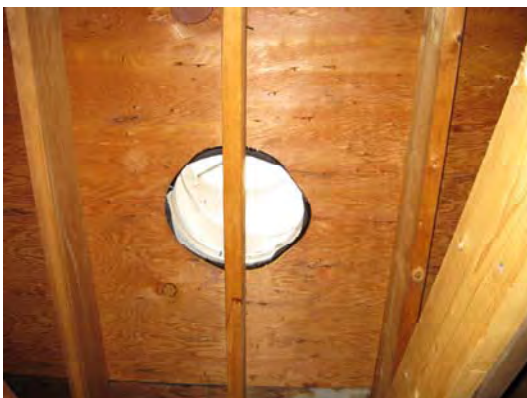
- Installed turbine vent - No staining on plywood
