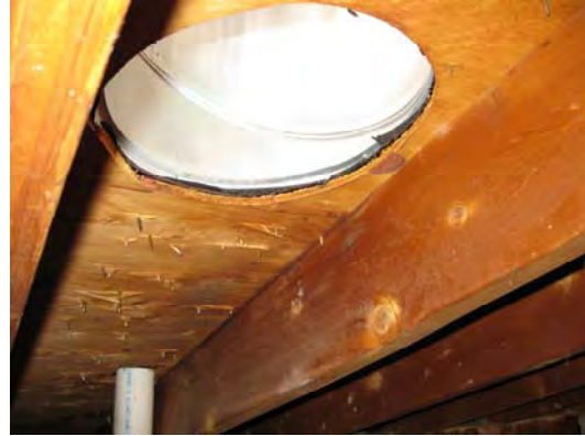
-Turbine vent, no plywood staining
