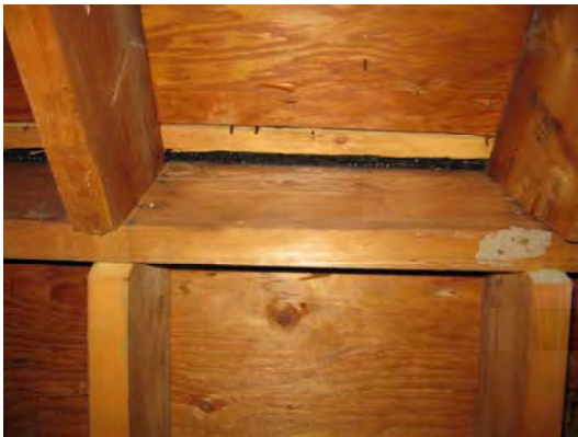
- Installed ridge vent
