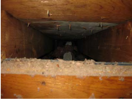
- Unblocked joist bay
