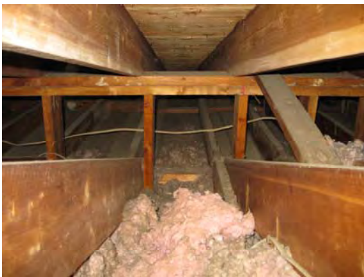
-Open joist bays
