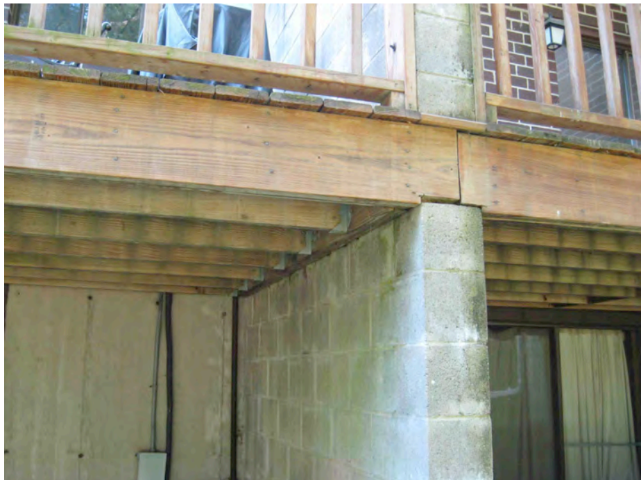
Photograph #5 – Wood Deck Joists Attached To CMU Wall
