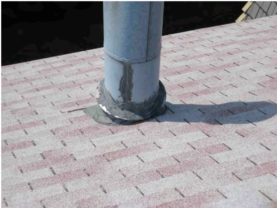
Photograph #9 – Mastic Repairs To Metal Furnace Vent
