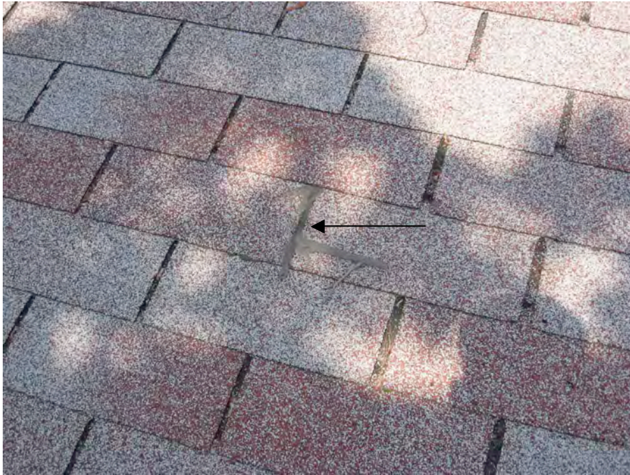
Photograph #8 – Sealant Repairs To Asphalt Shingles
