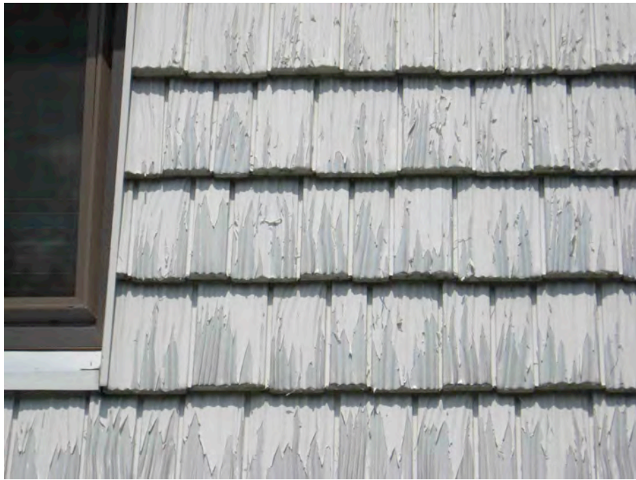
Photograph #14 – Finish Failure At Metal Panels
