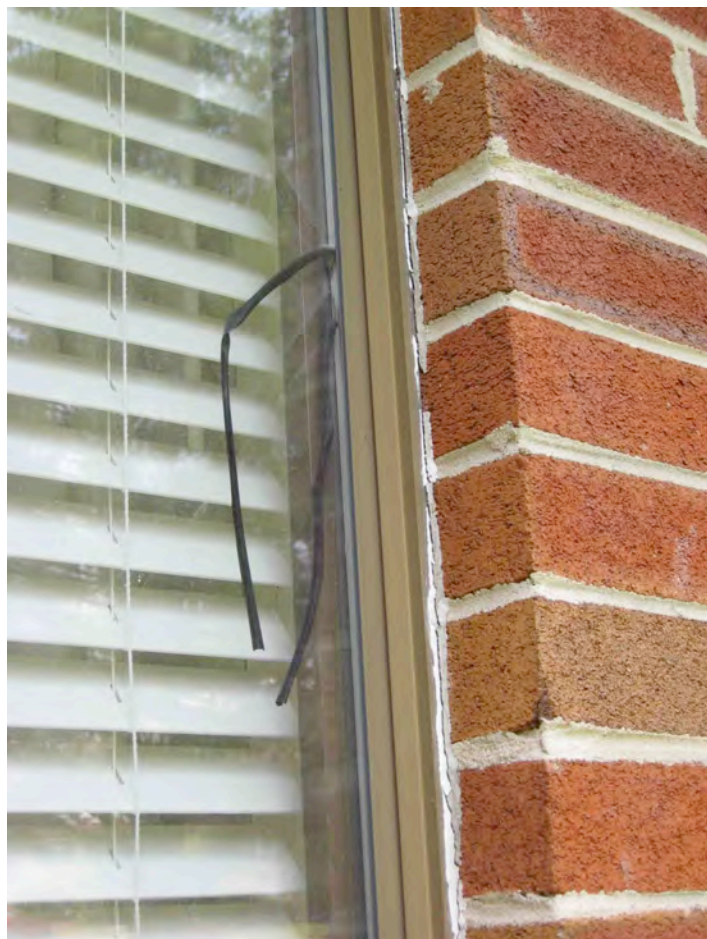
Photograph #14 – Finish Failure At Metal Panels
